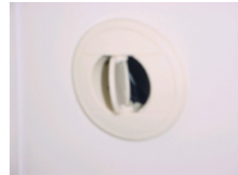
Air Conditioning Vents in the Mid Berth Cabin & Head
