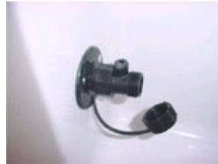
Lever on the washdown fitting is closed
