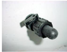
Lever on the aerator fitting is closed
