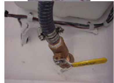
Seacock is shown in the closed position.
