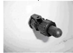
Lever on the aerator fitting is open
