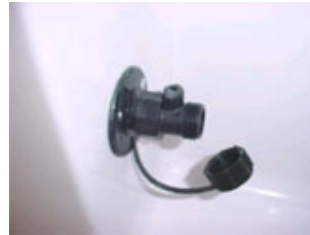
Lever on the washdown fitting is closed
