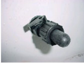
Lever on the aerator fitting is closed
