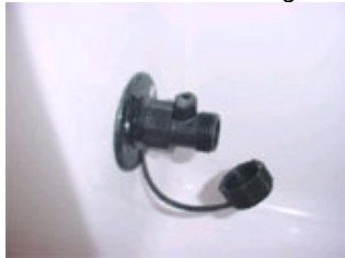
Lever on the washdown fitting is closed
