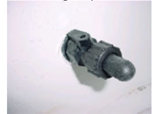
Lever on the aerator fitting is open
