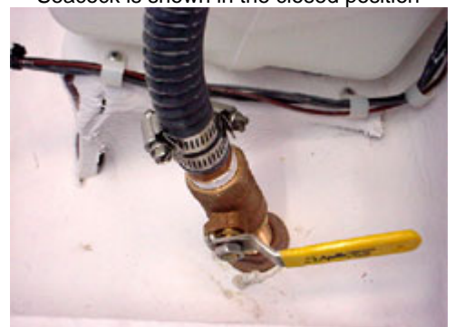
Seacock is shown in the closed position
