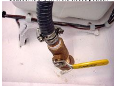
Seacock is shown in the closed position
