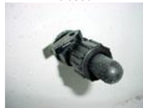
Lever on the aerator fitting is closed
