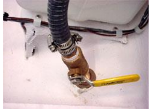
Seacock is shown in the closed position
