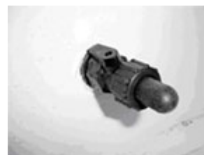
Lever on the aerator fitting is open
