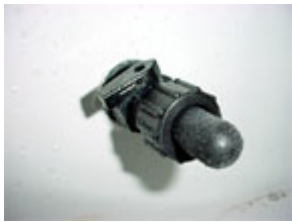
Lever on the aerator fitting is closed
