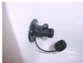
Lever on the washdown fitting is closed
