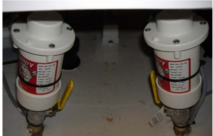
Lever on the aerator fitting is closed
