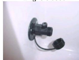
Lever on the washdown fitting is closed
