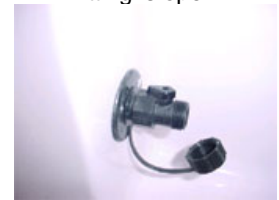
Lever on the washdown fitting is open
