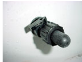
Lever on the aerator fitting is closed
