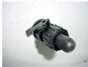
Lever on the aerator fitting is closed
