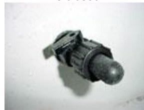
Lever on the aerator fitting is closed
