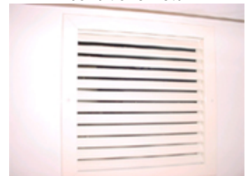
Air conditioner return
