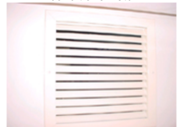
Air conditioner return
