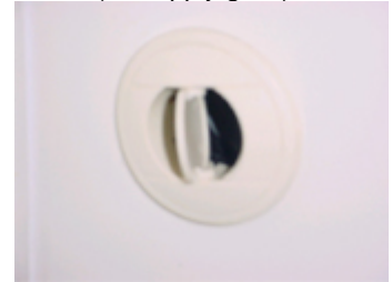
Air conditioning vent (air supply grille)
