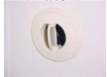
Air conditioning vent (air supply grille)
