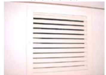
Air conditioner return
