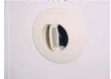
Air conditioning vent (air supply grille)
