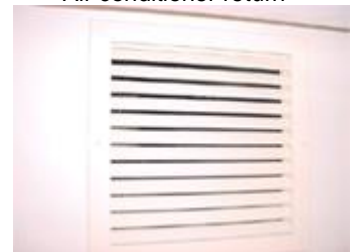
Air conditioner return
