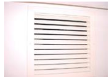
Air conditioner return
