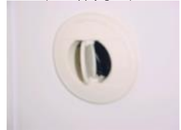
Air conditioning vent (air supply grille)
