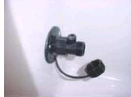
Lever on the washdown fitting is closed
