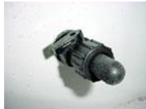
Lever on the aerator fitting is closed
