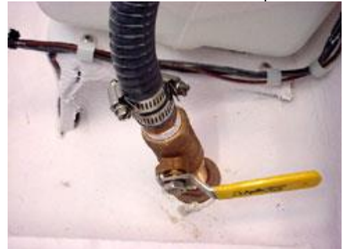
Seacock is shown in the closed position
