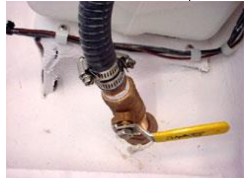
Seacock is shown in the closed position
