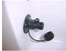
Lever on the washdown fitting is closed
