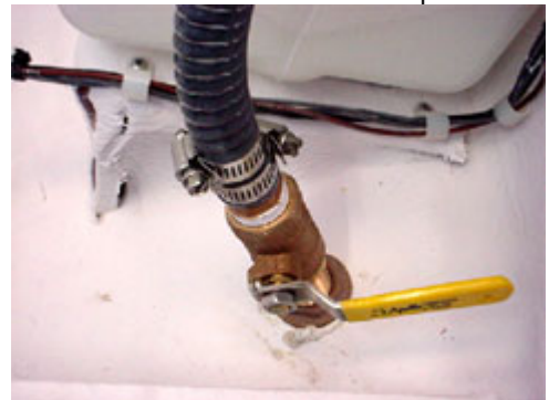
Seacock is shown in the closed position
