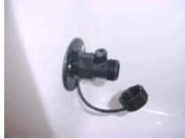
Lever on the washdown fitting is closed
