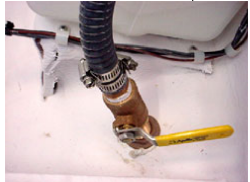
Seacock is shown in the closed position
