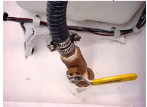
Seacock is shown in the closed position
