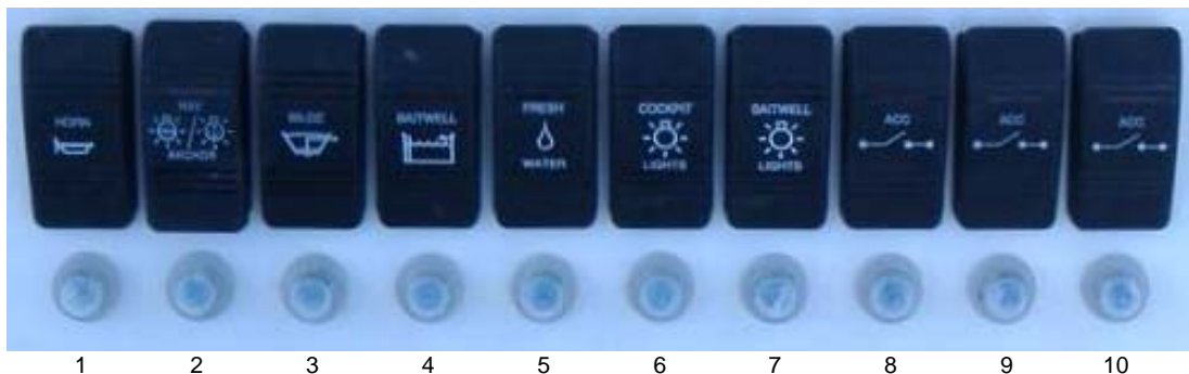
Circuit Breakers – On the switch panel below the individual switches
