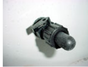
Lever on the aerator fitting is closed
