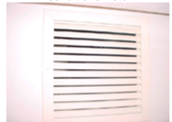
Air conditioner return
