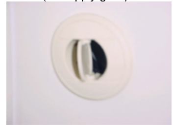
Air conditioning vent (air supply grille)
