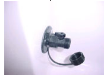
Lever on the washdown fitting is open
