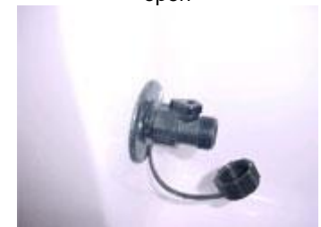
Lever on the washdown fitting is open
