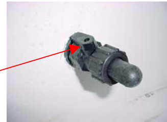
Lever on the washdown fitting is open
