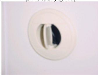
Air conditioning vent (air supply grille)
