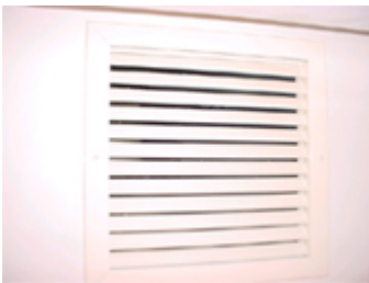
Air conditioner return
