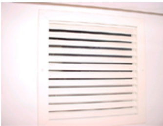
Air conditioner return
