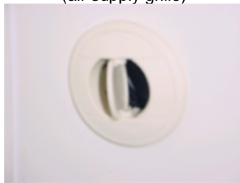
Air conditioning vent (air supply grille)
