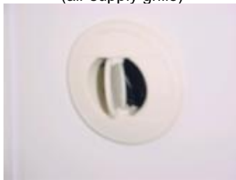
Air conditioning vent (air supply grille)
