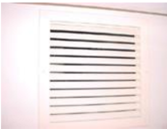
Air conditioner return
