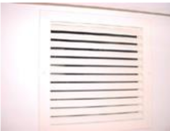
Air conditioner return
