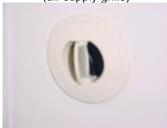
Air conditioning vent (air supply grille)
