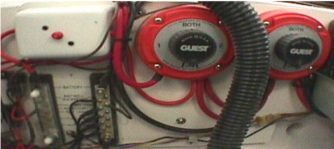
Bilge D/C Panel and Battery Selector Switches ^
