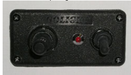
Remote Spot Light Control Panel
