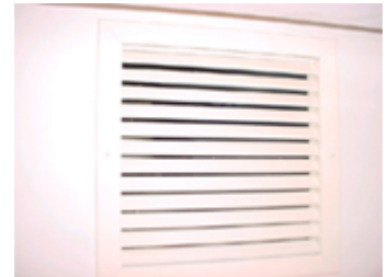
Air conditioner return
