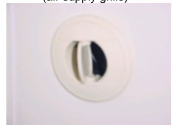
Air conditioning vent (air supply grille)
