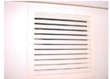
Air conditioner return
