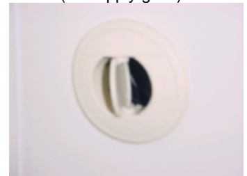
Air conditioning vent (air supply grille)
