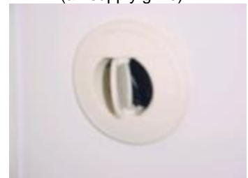
Air conditioning vent (air supply grille)
