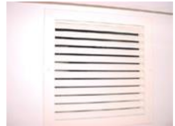
Air conditioner return
