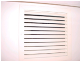
Air conditioner return
