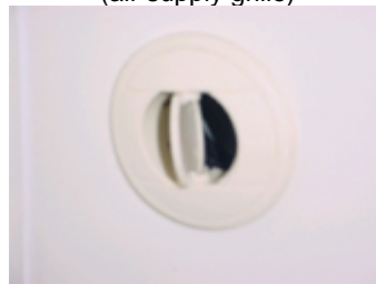
Air conditioning vent (air supply grille)
