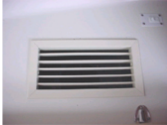
Air conditioning vent in the main salon
