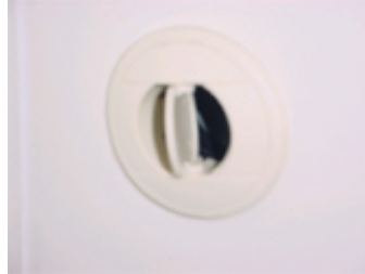
Air conditioning vents in the mid berth cabin and head
