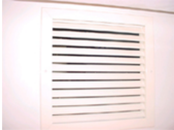
Air conditioner return on face of the V berth storage area
