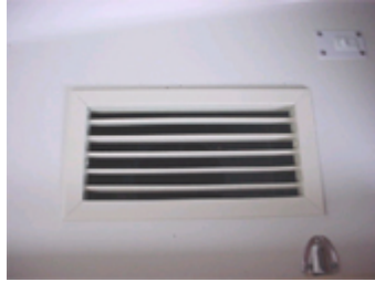
Air conditioning vent in the main salon
