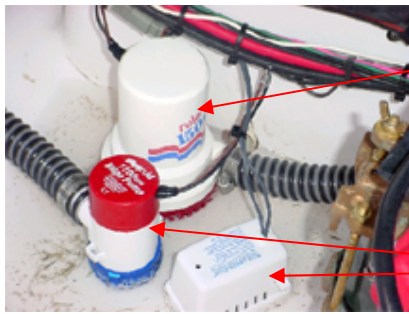
Bilge pump 2 (high water pump) Float switch is mounted aft of the port battery tray
