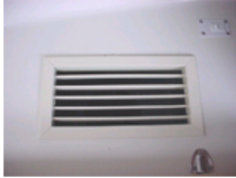
Air conditioning vent in the main salon
