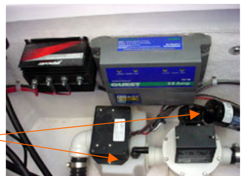
Aft Fish Box Pump and Collector Box
