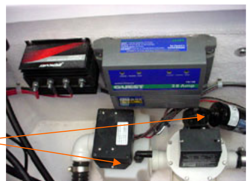
Aft Fish Box Pump and Collector Box
