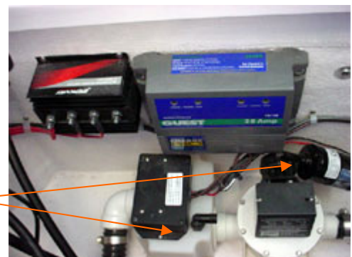
Aft Fish Box Pump and Collector Box
