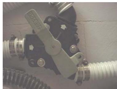
The “Y” valve for the Electric Head as shown here is set to use dockside discharge. Follow the arrows. Waste is going from the holding tank, to the “Y” valve and then upward to the waste outlet.
