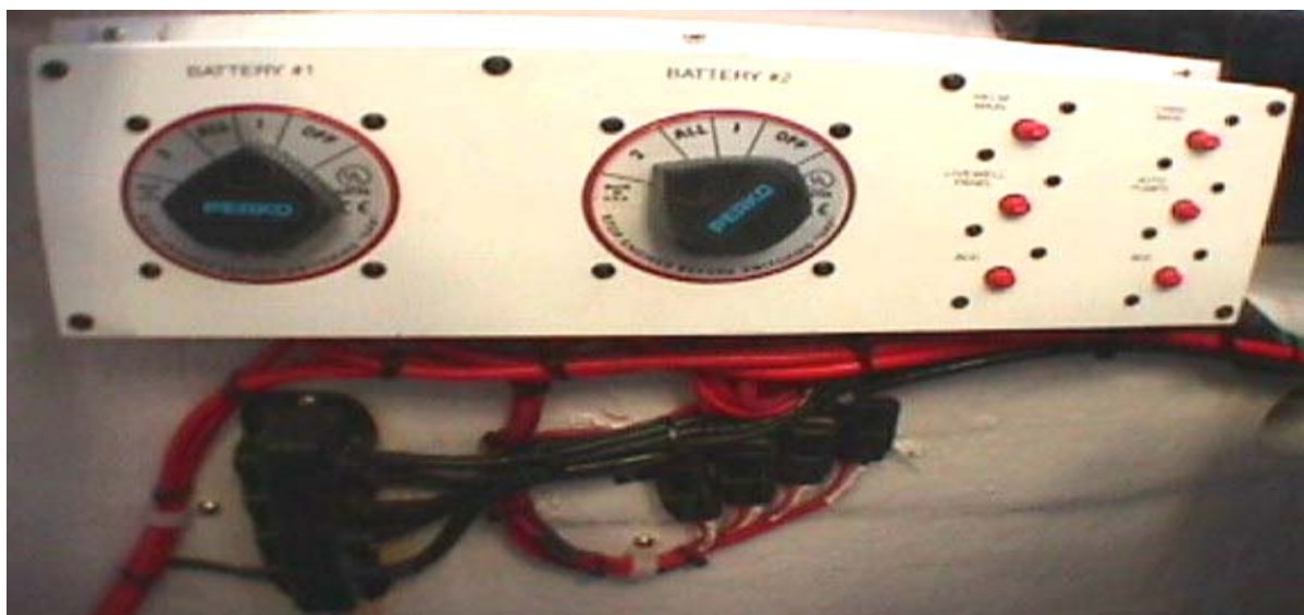
Bilge D/C Panel and Battery Selector Switches ^
