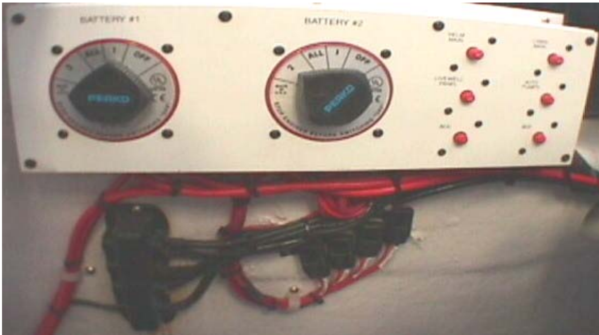
<fig. 5 – Bilge D/C Breaker Panel and Fuses>
