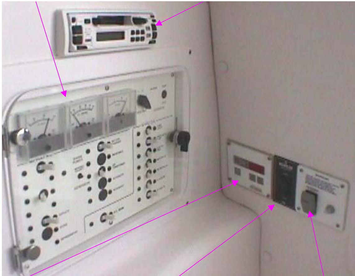
Air Conditioning Panel
