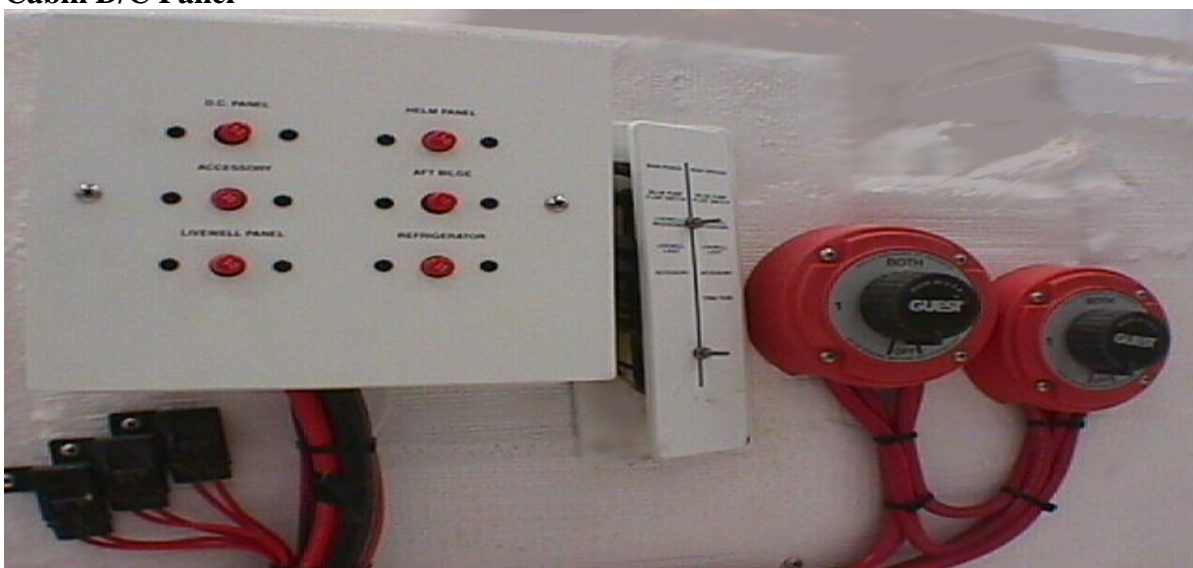
Bilge D/C Panel and Battery Selector Switches ^
