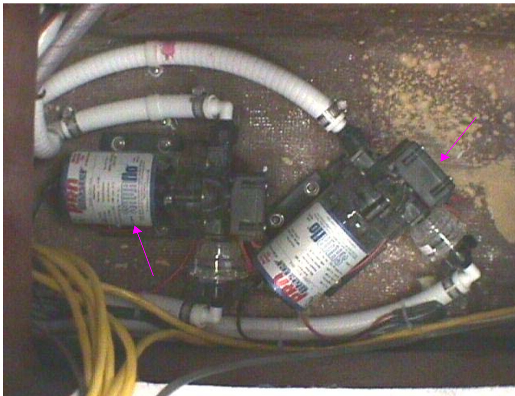
<fig. 6 – Fresh Water Pumps>
