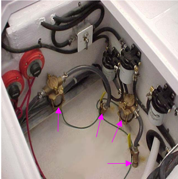
Air Conditioner and Generator Strainers and Seacocks
