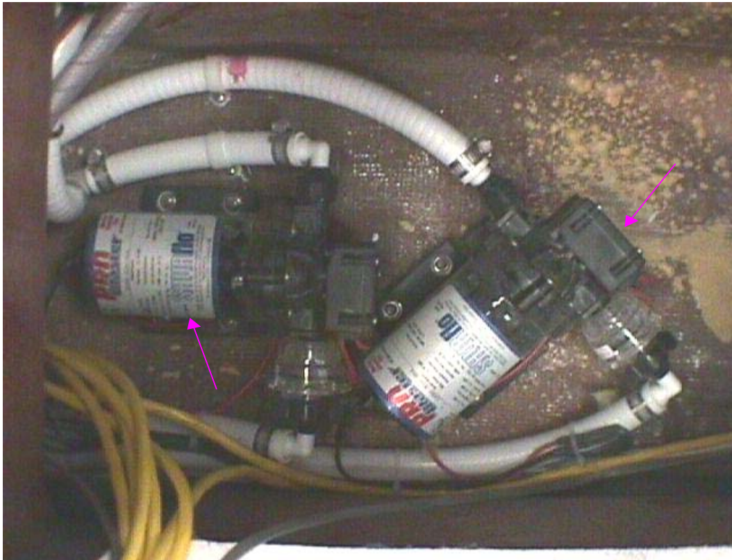
<fig. 6 – Fresh Water Pumps>
