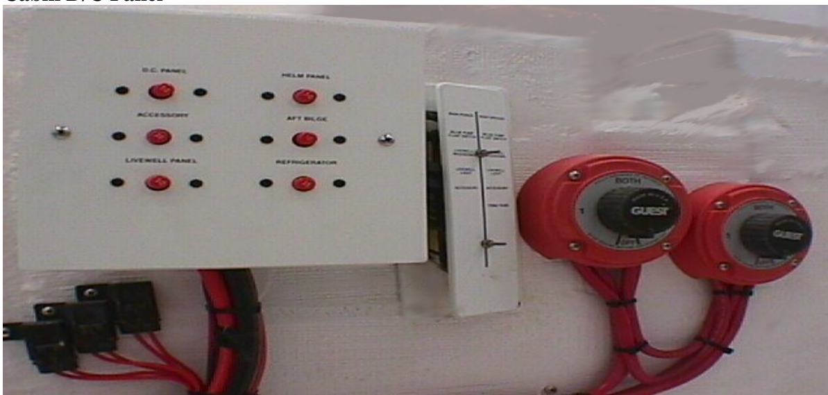
Bilge D/C Panel and Battery Selector Switches ^
