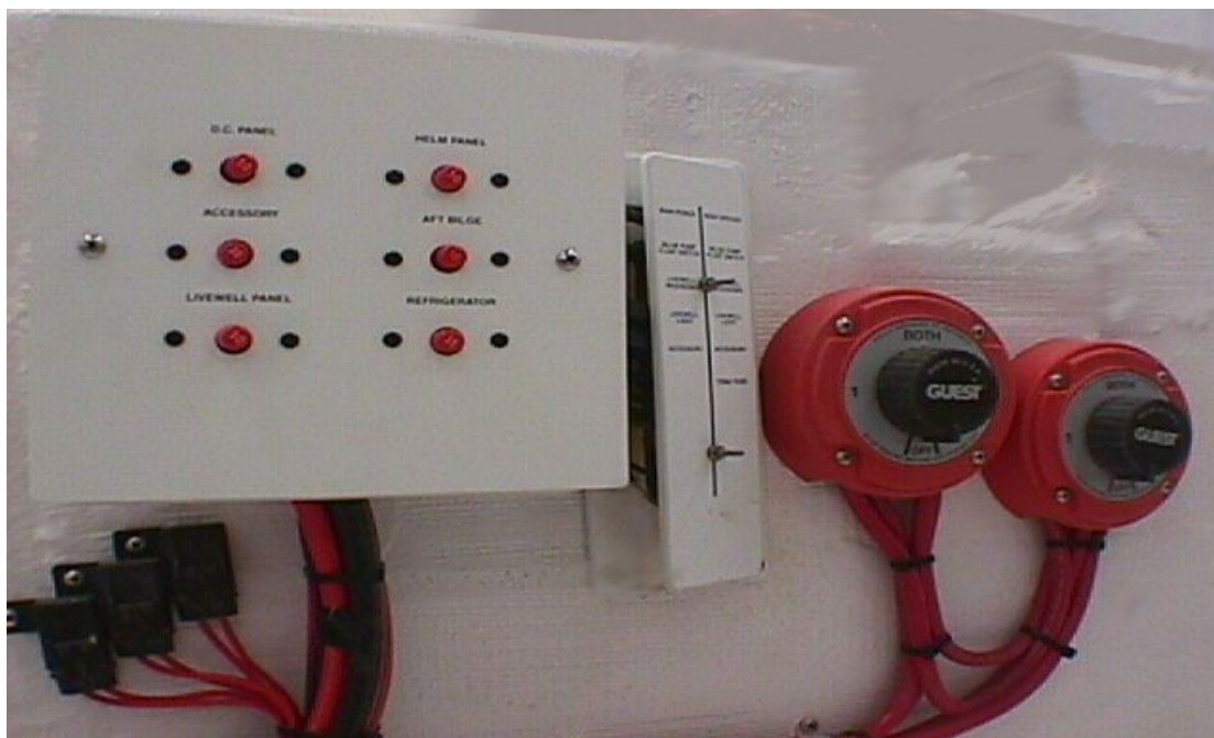
<fig. 5 – Bilge D/C Breaker Panel and Fuses>
