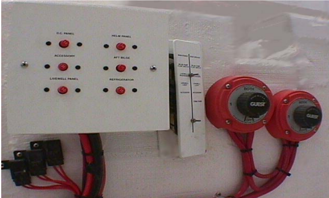
Bilge D/C Breaker Panel and Fuses
