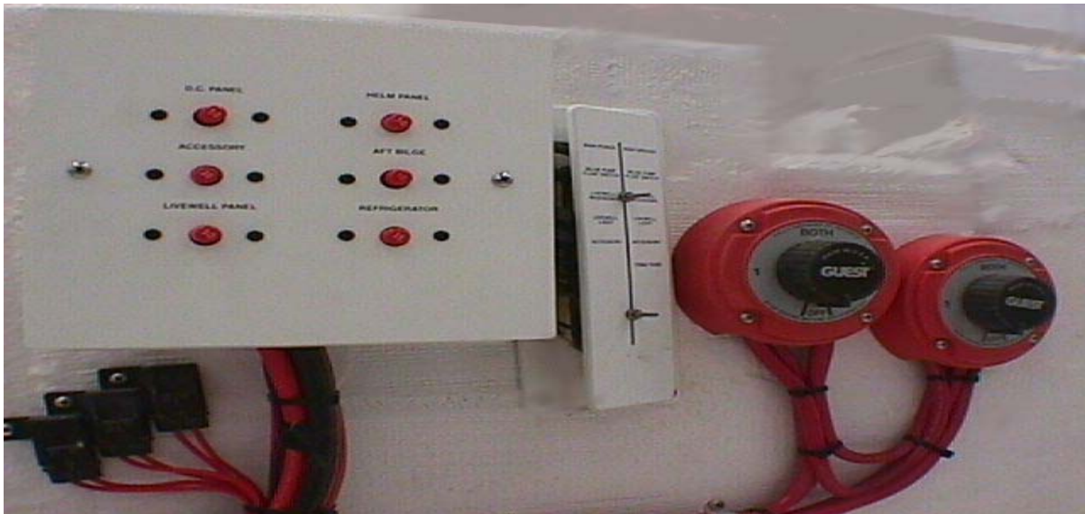
Bilge D/C Panel and Battery Selector Switches
