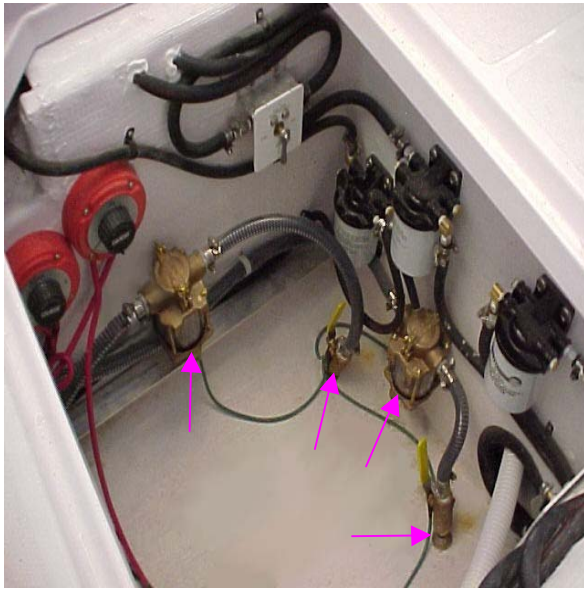
Air Conditioner and Generator Strainers and Seacocks
